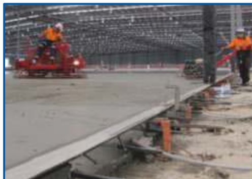
Concrete Casting Phase
