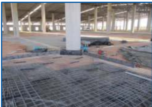
Steel Bar Preparation Phase
