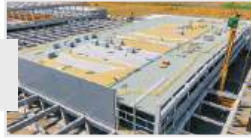
SYNERGY CONSTRUCTION Synergy Fabrika Projesi
